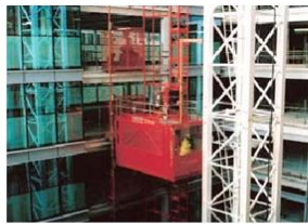
Rack and Pinion Drive Hoist
